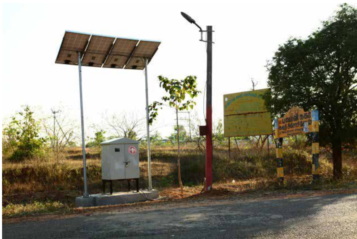
FIGURE 10: Solar street lighting
