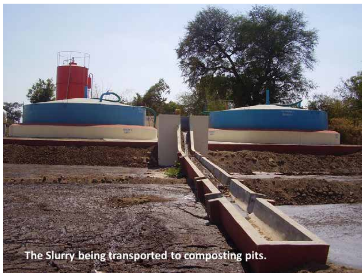
FIGURE 19: Community Biogas Plant at Bhintbudrak Village at Surat, Gujarat
